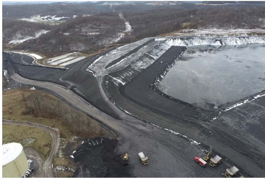
Figure 17-1: Downslope Coarse Refuse Placement on Leer South Impoundment (Photograph provided by Arch)
