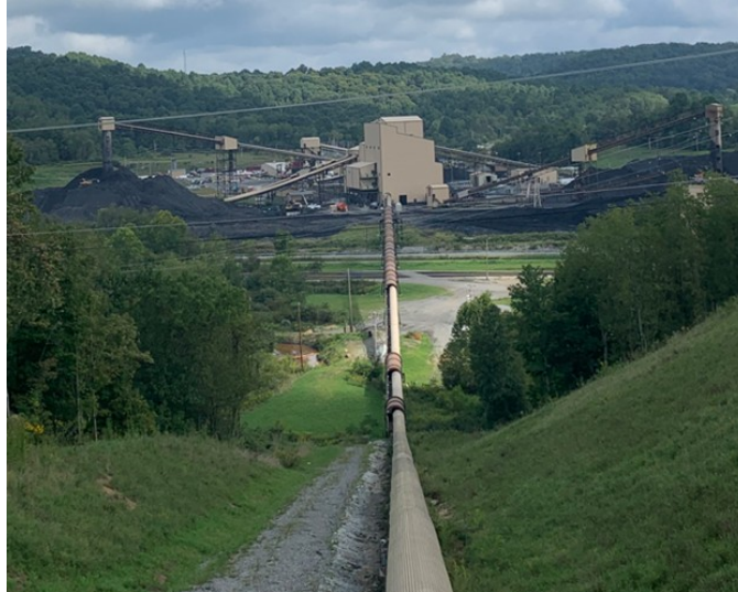
Figure 14-1: Leer South Preparation Plant as Viewed from Coarse Refuse Conveyor
