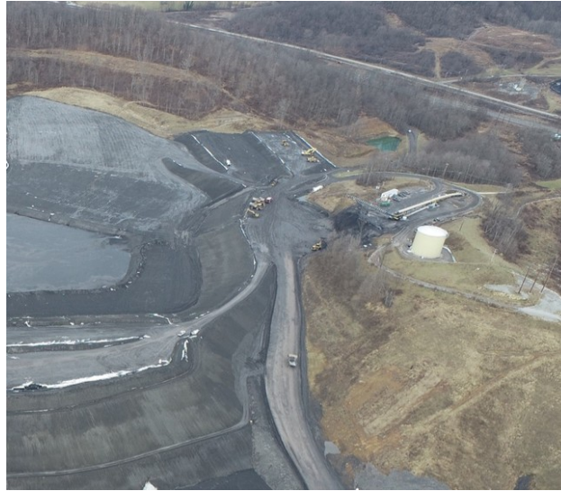
Figure 17-2: Coarse Refuse Stacker and Stockpile Area at Leer South (Photograph provided by Arch)
