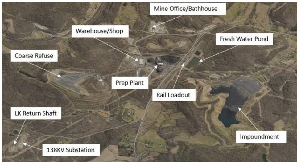
Figure 15-1: Leer South Surface Facilities
