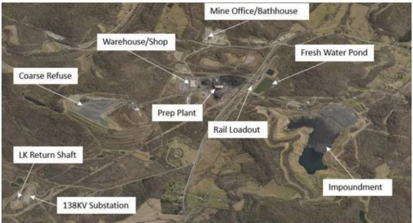
Figure 15-1: Leer South Surface Facilities
