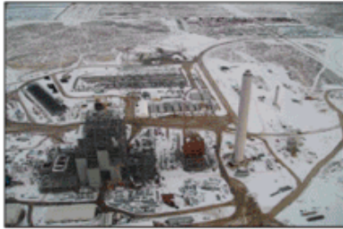
T.S. Power Boulder Valley (Nev.) 200 MW / Jan. 2010
